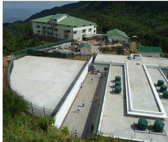
Figure 4. View of Montagne Posée Prison, Seychelles. Source: UNOPS/Trevor Sway
